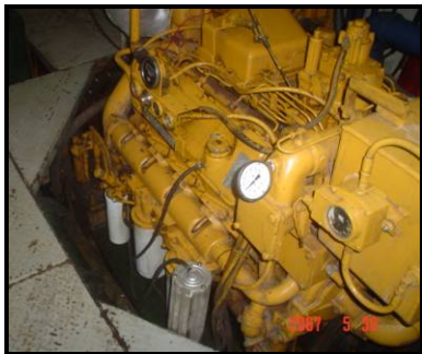
Trabold filter (Photo courtesy of Ecoventura)
